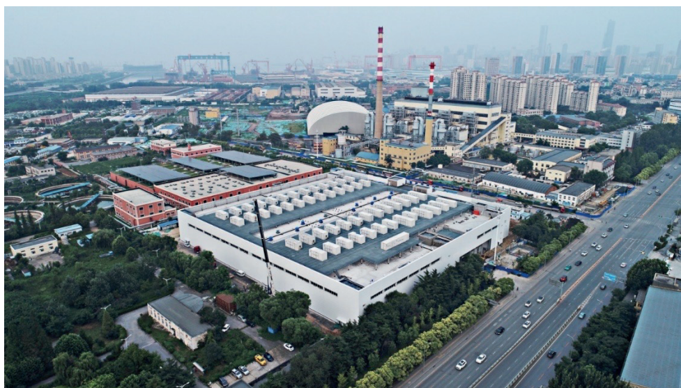
Figure 1 – Dalian Constant Current Energy Storage Power Station Co., Ltd., featuring a battery energy storage system
