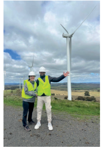
Capital Wind Farm
